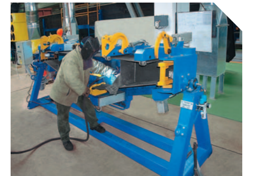
Front beams assembly stand
