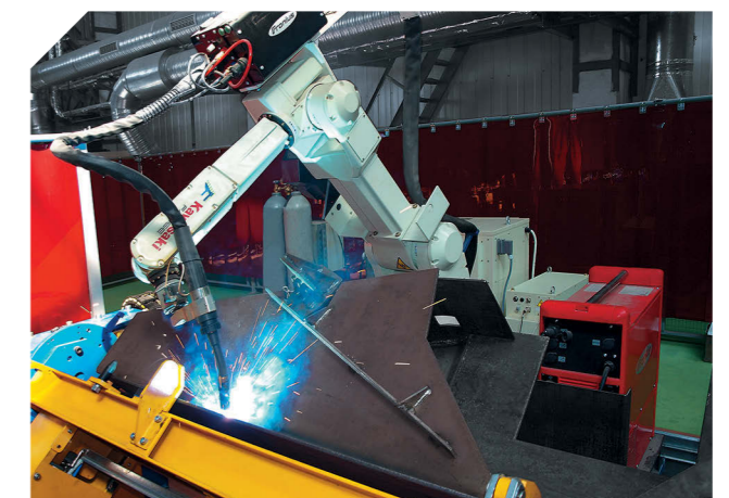
Robotic welding of cross bearers
