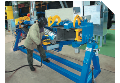
Front beams assembly stand
