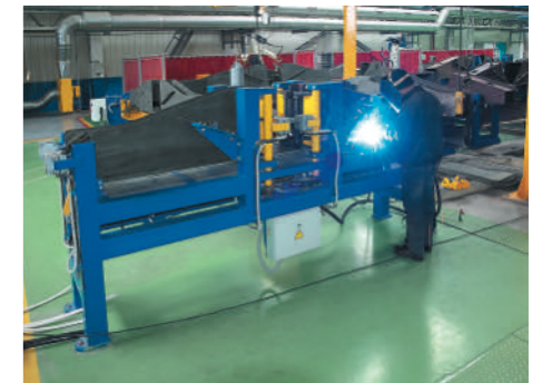
Intermediate beams assembly and welding line
