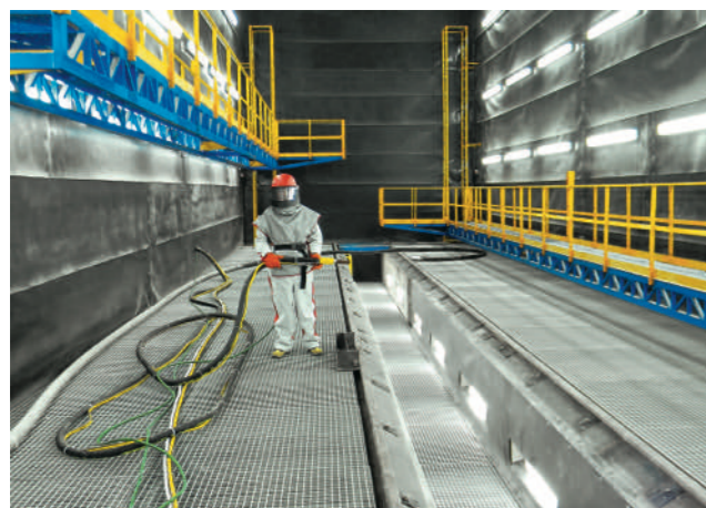
Shotblasting chamber for cars
