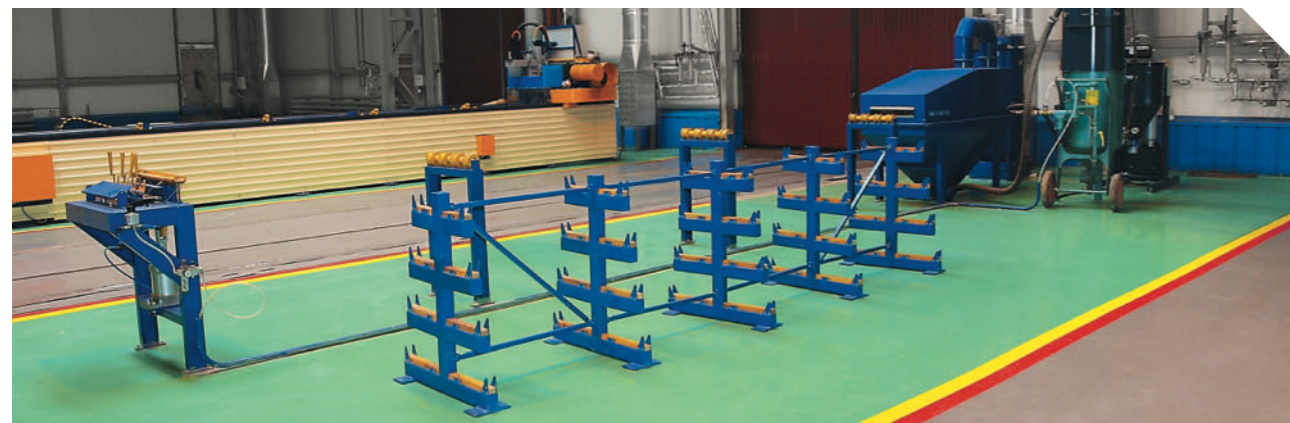
Shotblasting plant for cleaning of pipes inner surface
